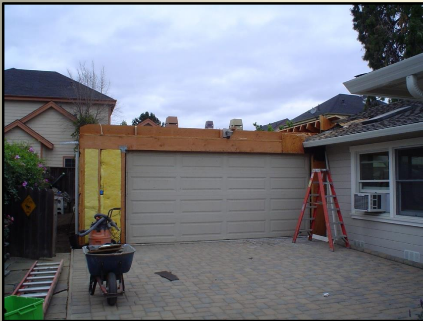
Original garage with roof removed
